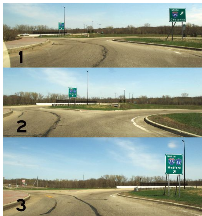
Figure 3. A sequence of signs within a roundabout indicates how the proximity of signs to a decision point and the location of signs relative to a decision point can lead to confusion.
